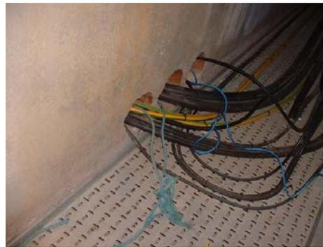
**Figure A-4 - Power and control cables share ducts**
