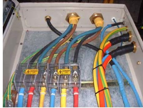
**Figure A-2 - Junction box connections**
